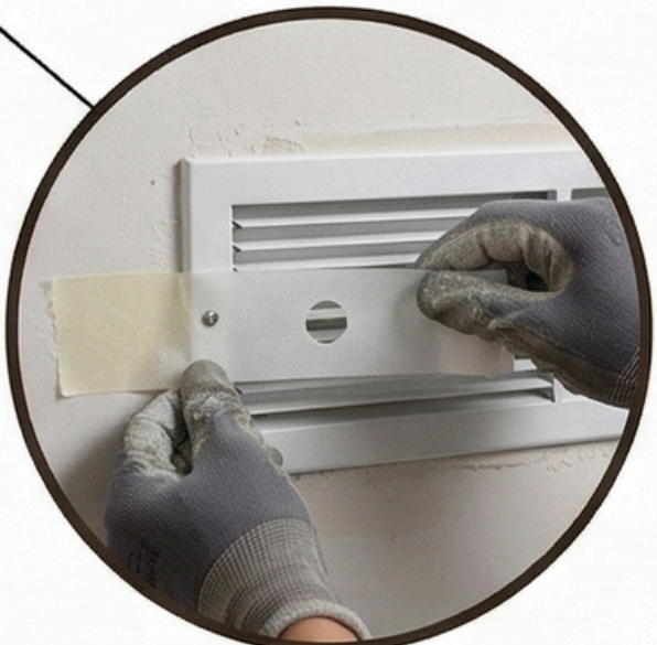
HVAC MASKING TAPE
